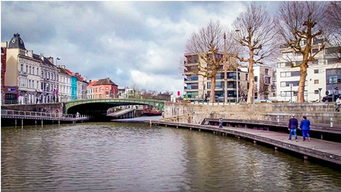
Bridge Contributiebrug on the entrance to the city of Ghent (Belgium)
