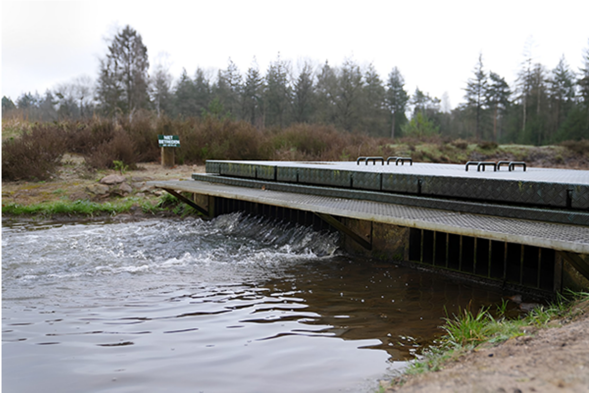
Intake area for the infiltration at the infiltratiegebied Koekenberg, near the Osssenweg Epe (Netherlands)
