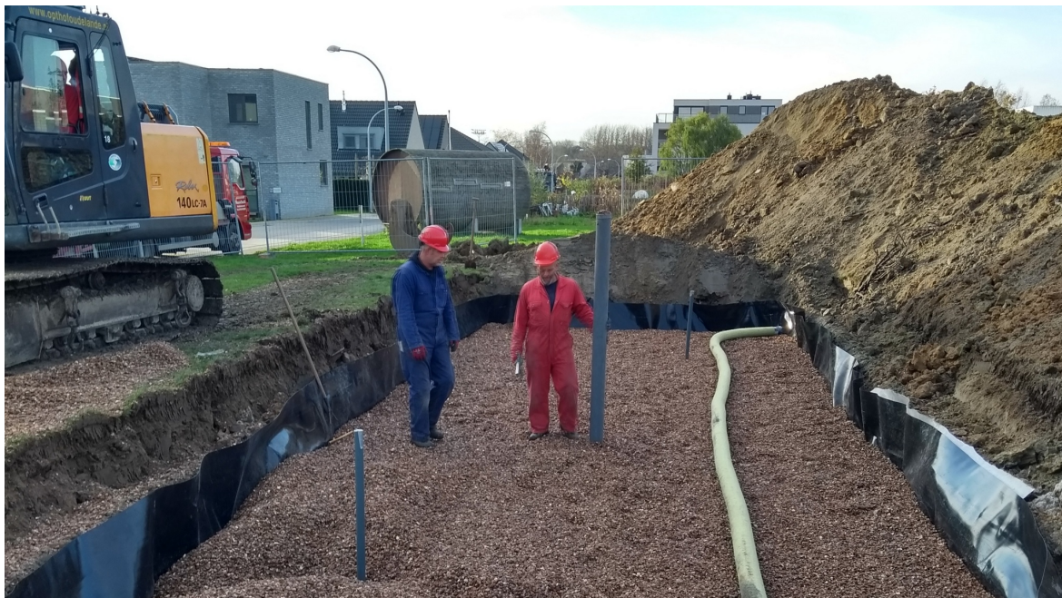
Construction of the shell-based system in Wetteren, Belgium. © Birgit De Bock, 2020
